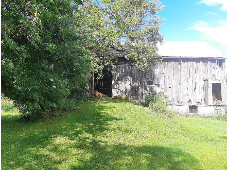
Photo 5 View of the on-site barn, September 7, 2022.
