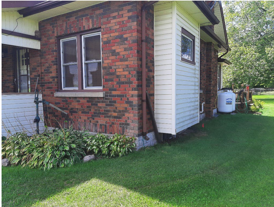
Photo 1 North side of the on-site residential dwelling, September 7, 2022.
