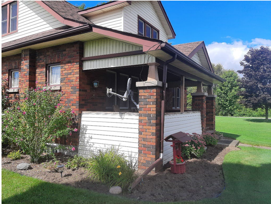
Photo 3 East side of the on-site residential dwelling, September 7, 2022.
