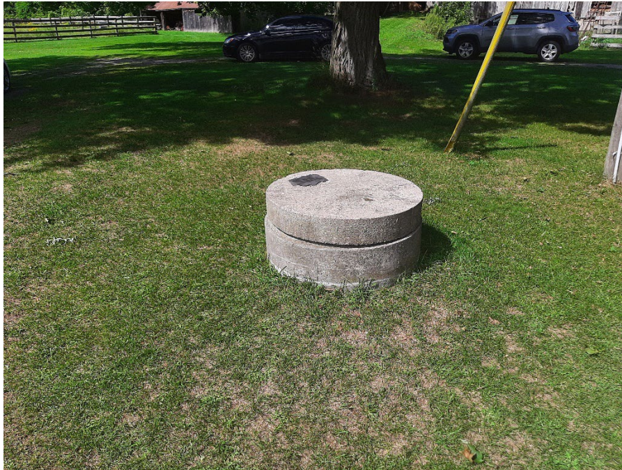
Photo 7 Dug well northwest of the on-site residential dwelling, September 7, 2022.
