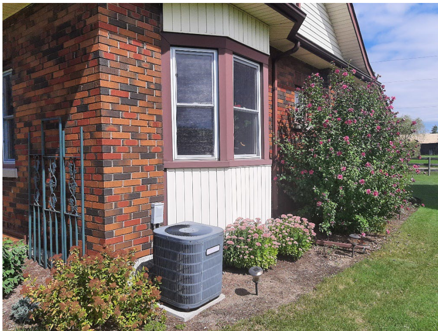
Photo 2 South side of the on-site residential dwelling, September 7, 2022.
