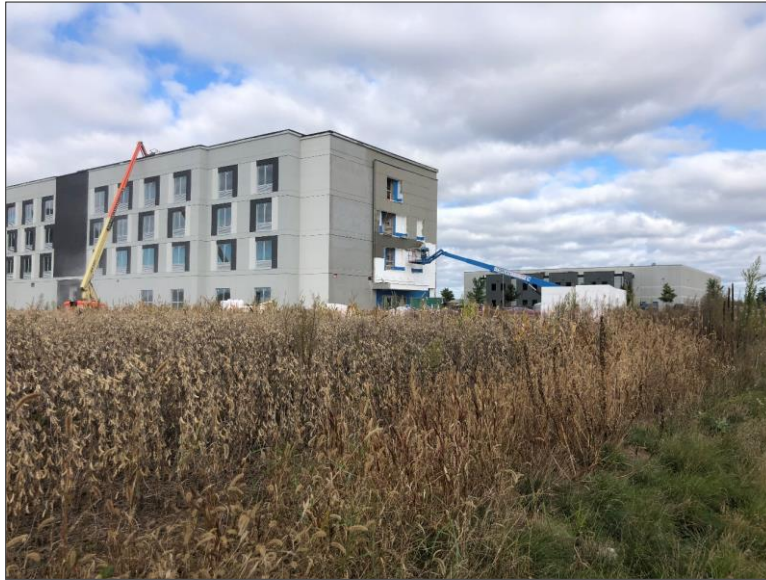
Photo 3 – Properties located north of the Site.
