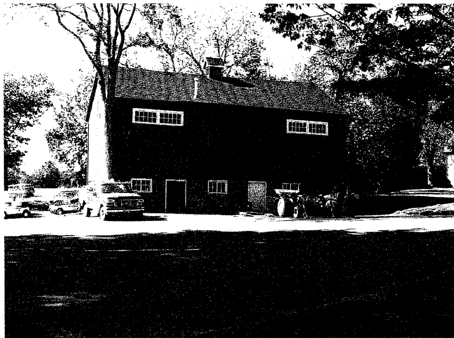
Photograph 4: Looking northerly at the works barn. Above ground hydraulic hoist is located beside the tractor.
