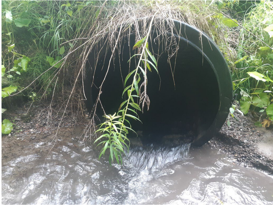
Photo 7 Culvert outlet at northern Mill Street crossing, July 2021.
