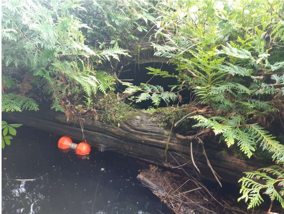
Photo 5 Culvert inlet on Mill Street, southern crossing, July 2021.
