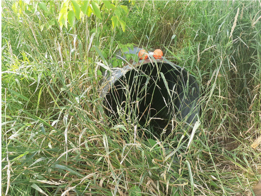
Photo 3 Culvert inlet (embedded) on north side of Ganaraska Road, July 2021.
