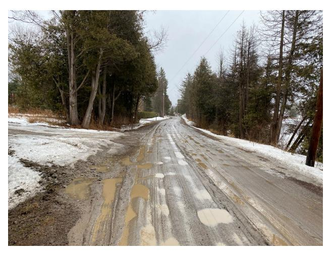
Monument conducted a topographic survey of Mill Street in September 2022. The extent of the survey was carried from the Ganaraska Road intersection for a total length of 1050m north past the extent of the Mistral property. The survey revealed a gravel driving platform of roughly 5.5m with very shallow ditching (~0.3m) along the east side of the roadway. The existing alignment is illustrated in the attached drawings (06).
