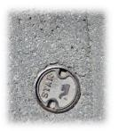
A **main valve** controls the flow of water passage throughout the water distribution system and can be used to isolate areas for maintenance or replacement.
