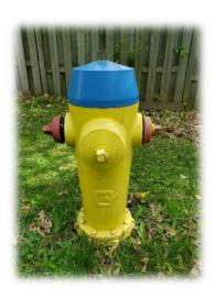
A hydrant is a visible fixture placed outside a building, parking area, industrial area, or roadside that is connected to the municipal or a private water service network. They are used for flushing the mainline; creating a scouring action to clean the line. Fire hydrants are designed to instantly provide the water required by fire fighters to extinguish a fire.
