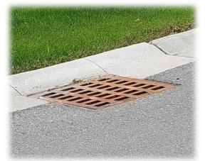
A **catch basin** is, in other words, a storm drain. They are used to redirect water to prevent flooding and are common on public streets. Catch basins collect rainwater or melted snow and transport it to an outfall reservoir.
